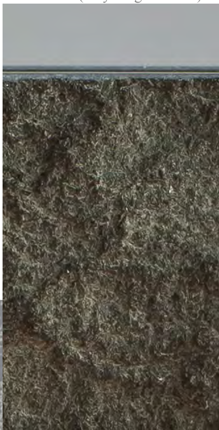
*Rockfaced (very rough surface)
